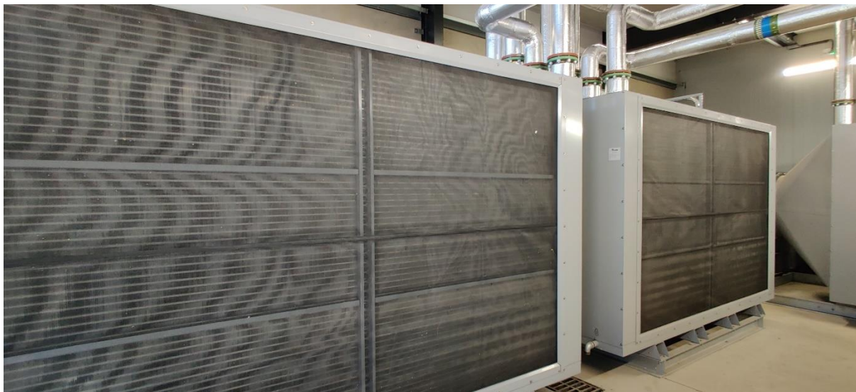
Figure 6: Heat exchangers in front of floor dryer intake fans. In this ground source heat pump system has a ground loop heat exchanger directly in front of the hot water heat exchanger. This condenses water vapour drying the air before heating. De humidifying in this manor leads to a greater humidity deficit than is achieved by heat alone. Note the drain on the heat exchanger unit for condensed water.
